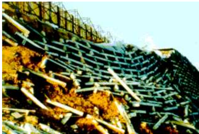
Figure 2-8 Example Condition for Strength Limit State Evaluation
